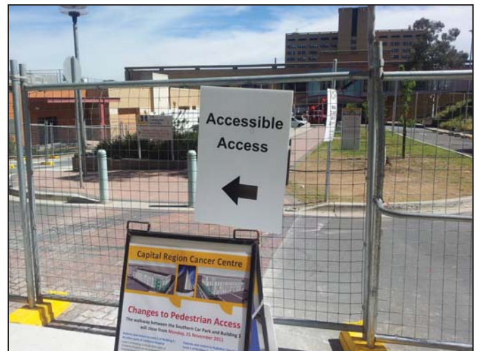
Construction site at Canberra Hospital. Observed by Charles Storey
